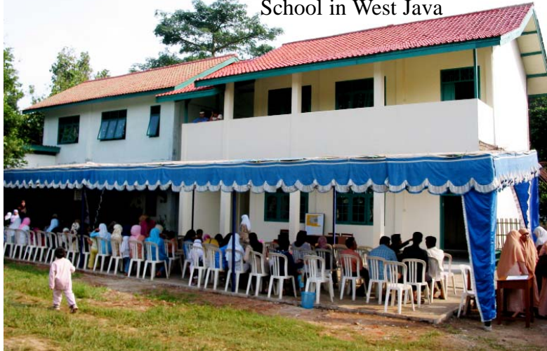
The new addition of a Primary School in West Java
